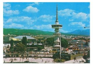
The tower was constructed on three vertical load-bearing components made of reinforced concrete. Its total height, including the antenna, is 72.4 meters, thus creating a strong landmark. The horizontal components which appear as polygonal surfaces draw morphological references from the elements of wireframe and framework.. High quality in terms of construction of the building allowed for the minimum utilization of the structural advantages that reinforced concrete offers.
